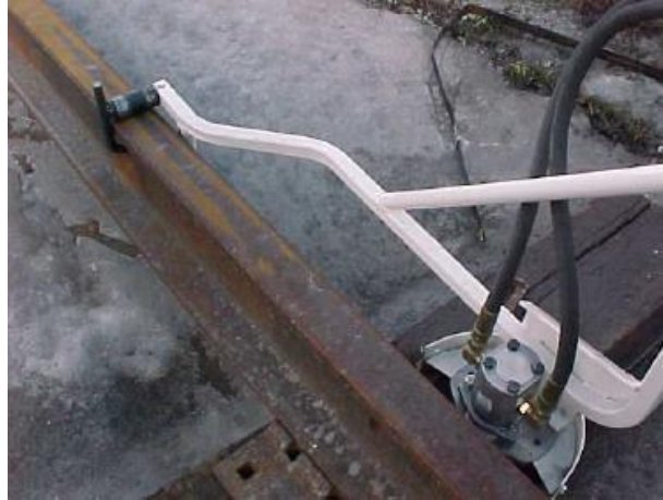
Web Grinder on the rail.
